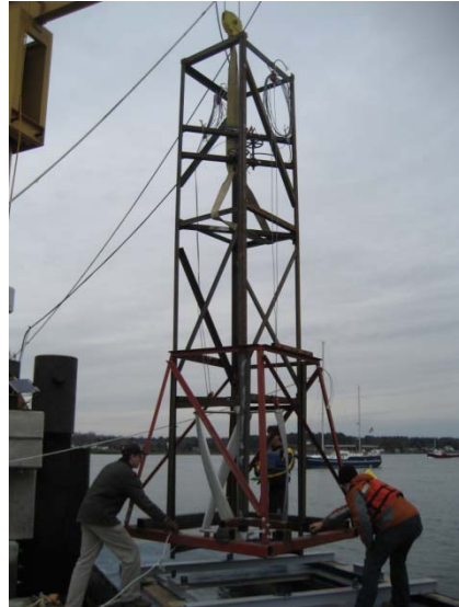
Figure 14: Lowering Cage and Derrick Onto Platform
