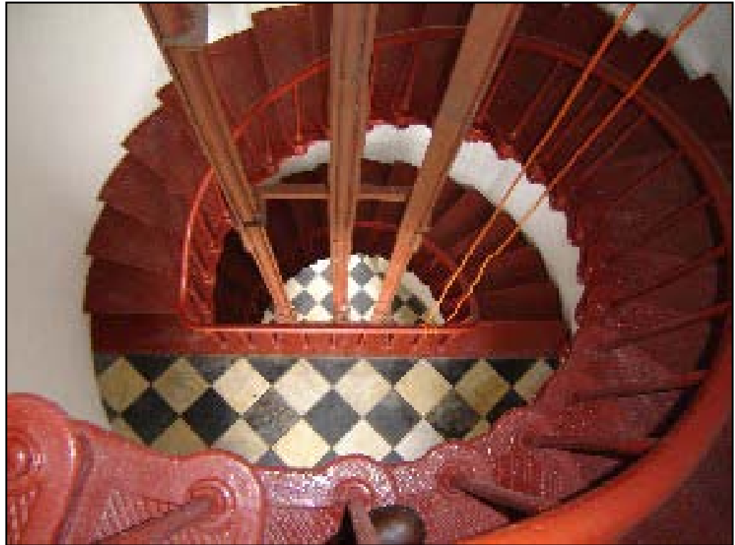
Staircase, Hatteras Light (photo NPS)
