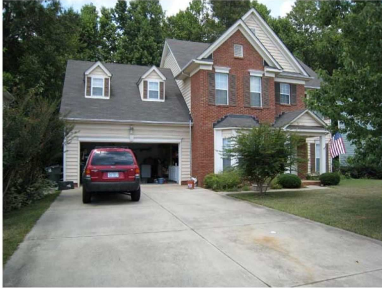
Figure 9: Test home for preliminary FDD experiments with HVAC.
