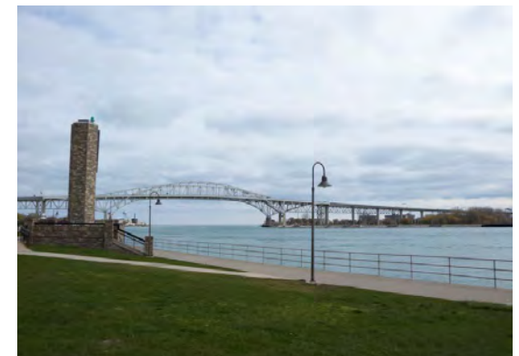
View of Blue Water Bridge. Elizabeth Durfee
