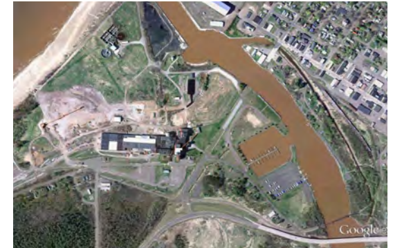
Smurfit-Stone Co. paper plant. Google Maps
