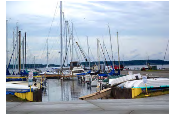
Docks and ramp at Torrensen Marine. Elizabeth Durfee
