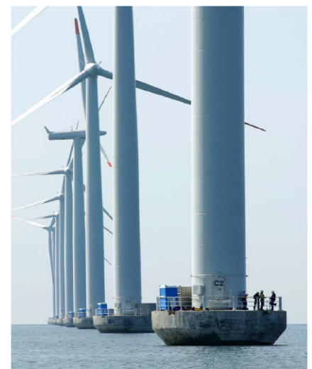
Figure 4. The foundations at the Nysted offshore wind farms are equipped with inverted ice-breaking cones.
