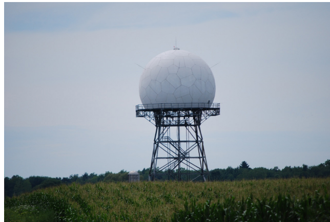
Figure 1: FAA's ARSR radar system (Photo: J. VanderMolen).
