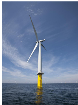
Figure 5: Offshore wind turbine with base painted yellow up to 50 feet above the highest astronomical tide (Photo: DONG Energy).
