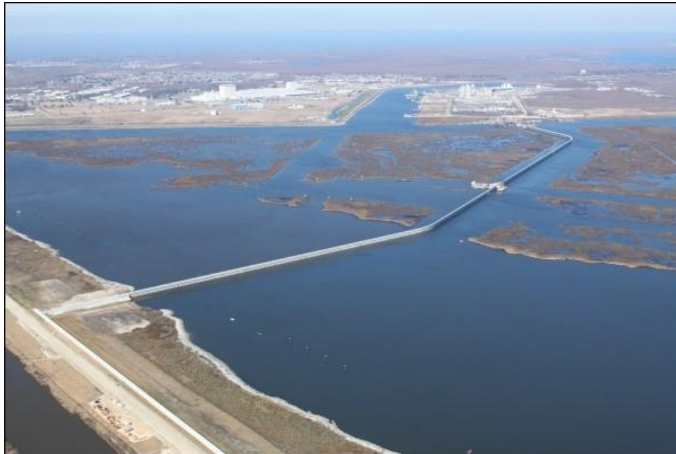
Figure 40: IHNC surge barrier aerial photo (source: google images)
