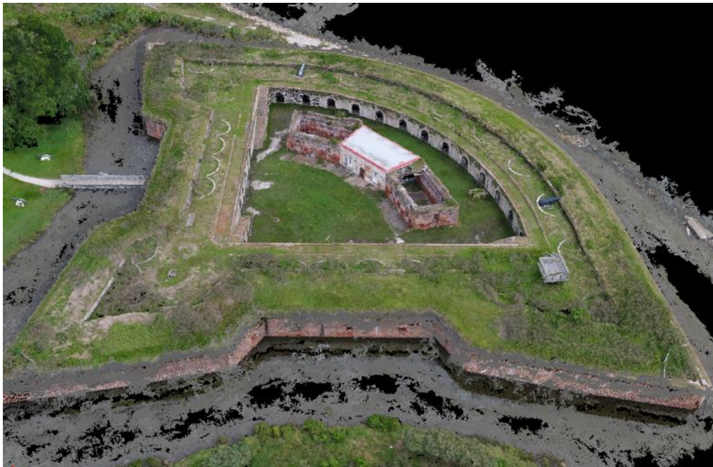
Figure 35: Aerial image of the project site
