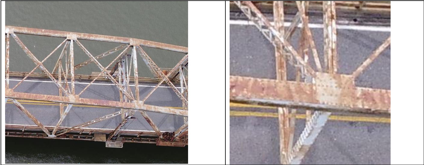
Figure 27: Close up image of bridge component
