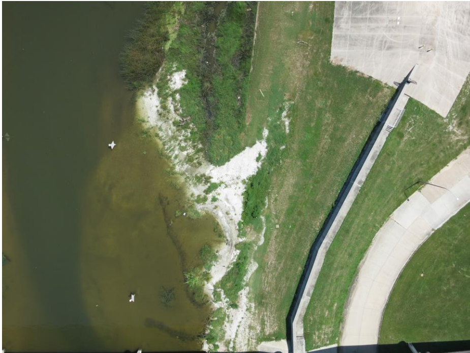
Figure 19: Aerial image of the project site
