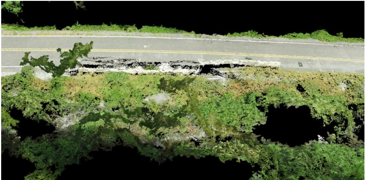
Figure 22: Aerial image of the project site
