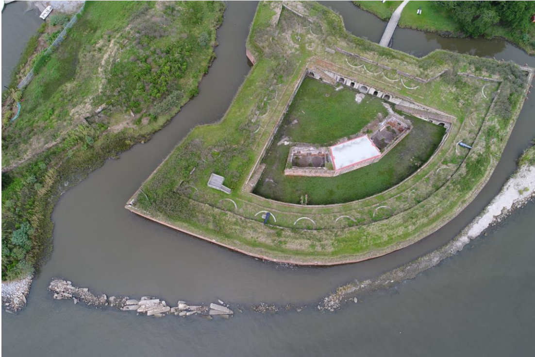
Figure 36: Aerial image of the project site
