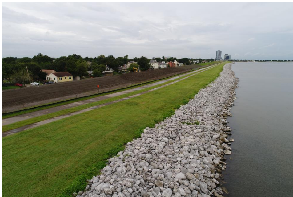
Figure 31: Aerial image of the project site
