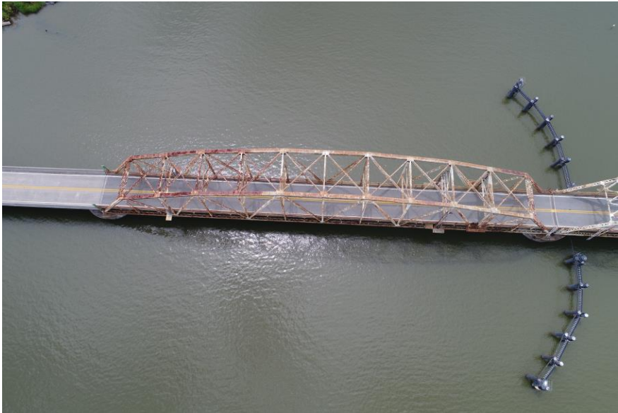
Figure 26: Aerial image of the project site
