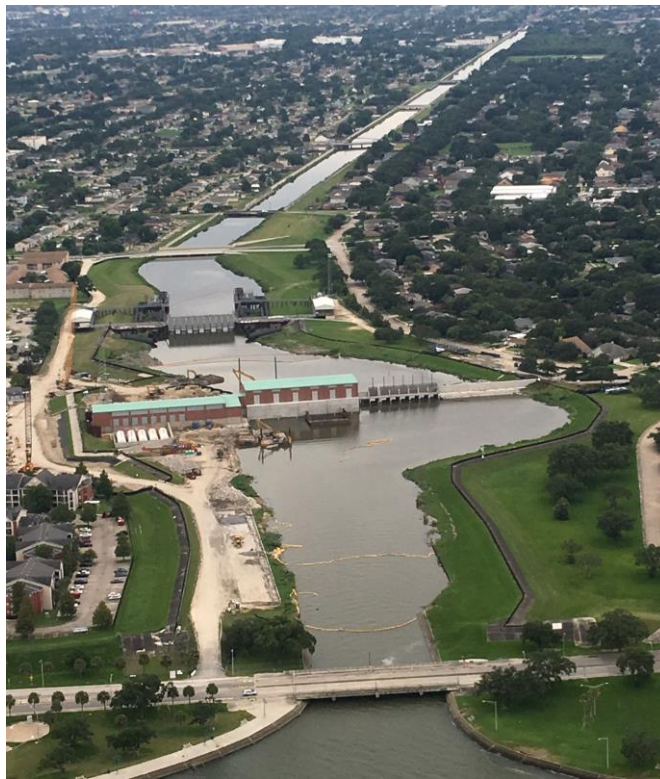
Figure 42: Canal and pump station along Lake Pontchartrain
