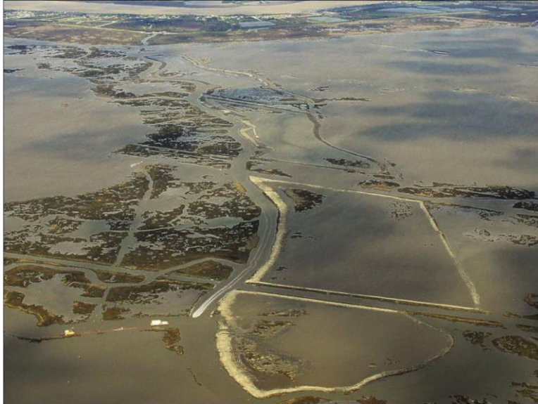
Figure 43: Marsh creation project in progress (source: Louisiana CPRA)
