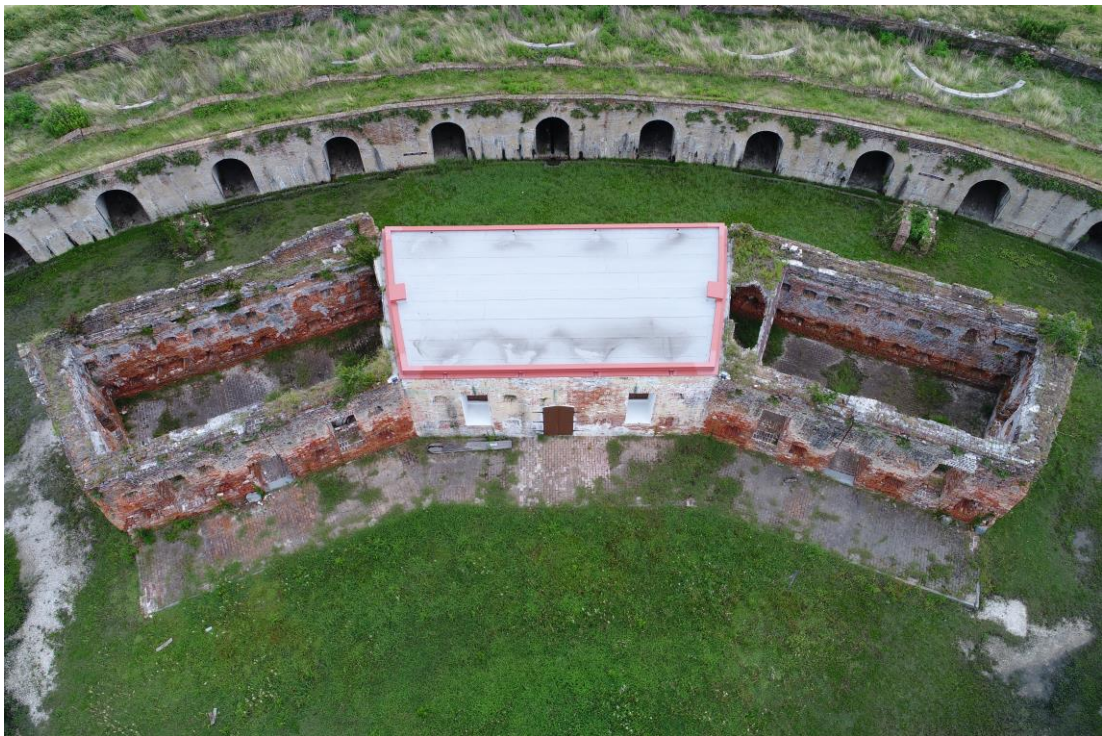
Figure 37: Aerial image of the project site
