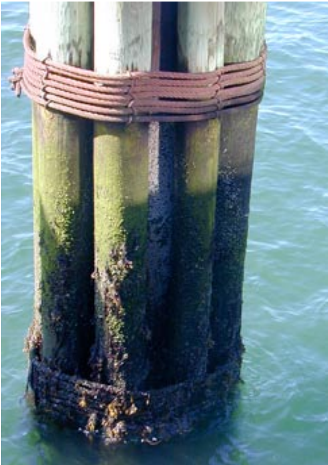
Wooden piling in Boston Harbor, Massachusetts, colonized by a fouling community. Ben Fertig
