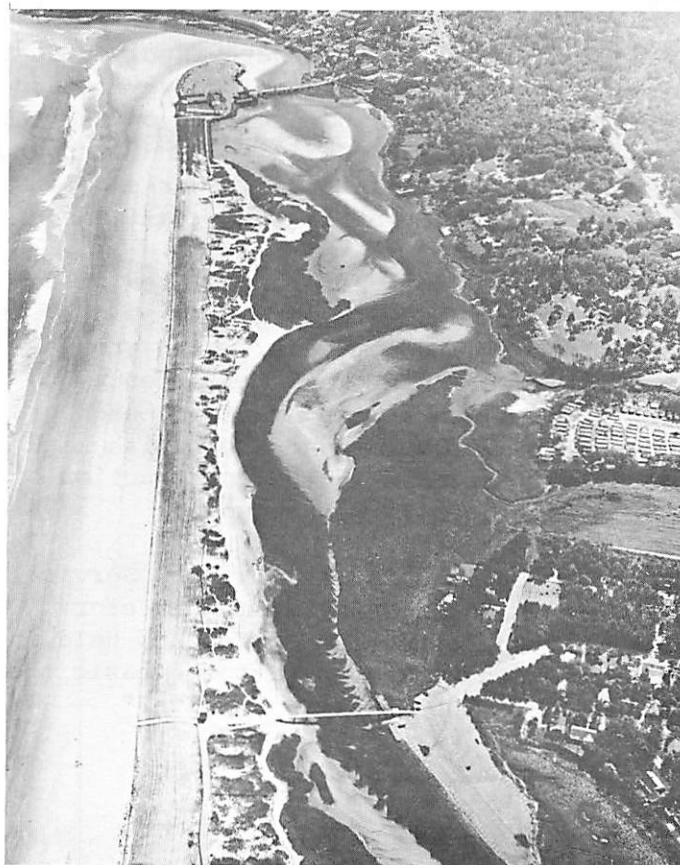
September, 1975: The completed dike is shown.
