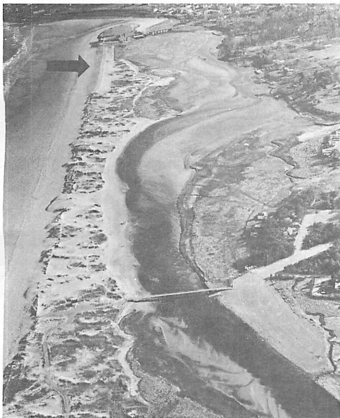
April, 1974: Only the first section of dike (arrow) had been constructed.
