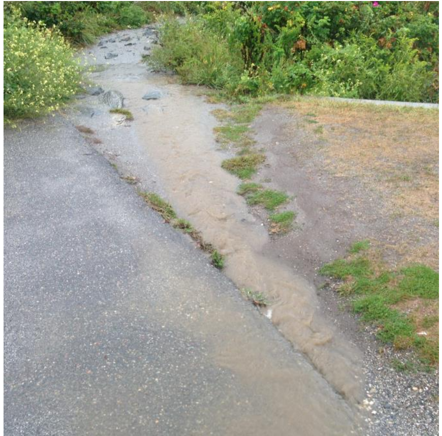
Photos this page: Sediment from Marine Avenue runoff flows directly into Rhode Island Sound along the Cliff Walk near Belmont Beach, Newport.
