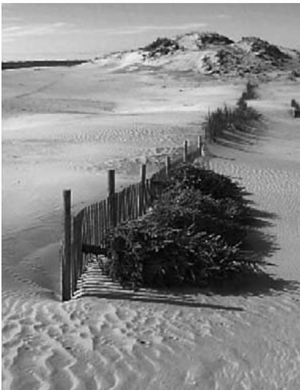
Discarded Christmas trees in a spur configuration enhance sand fence (image: Mitasova et al., 2005).
