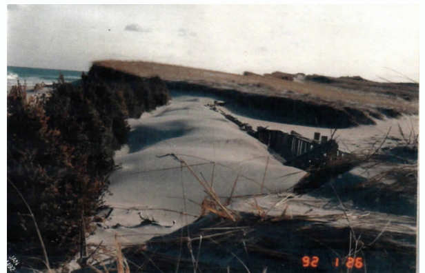
Sand fences enhanced by discarded Christmas trees to mimic a double row of sand fence. Image from 1992 courtesy of Massachusetts Beach Buggy Association.
