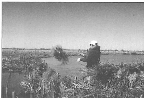
A Louisiana worker tosses another tree along a fence line, to slow erosion and help build and protect vulnerable areas within the marsh. The Christmas Tree Fence Project is operated by the Louisiana Department of Natural Resources.
