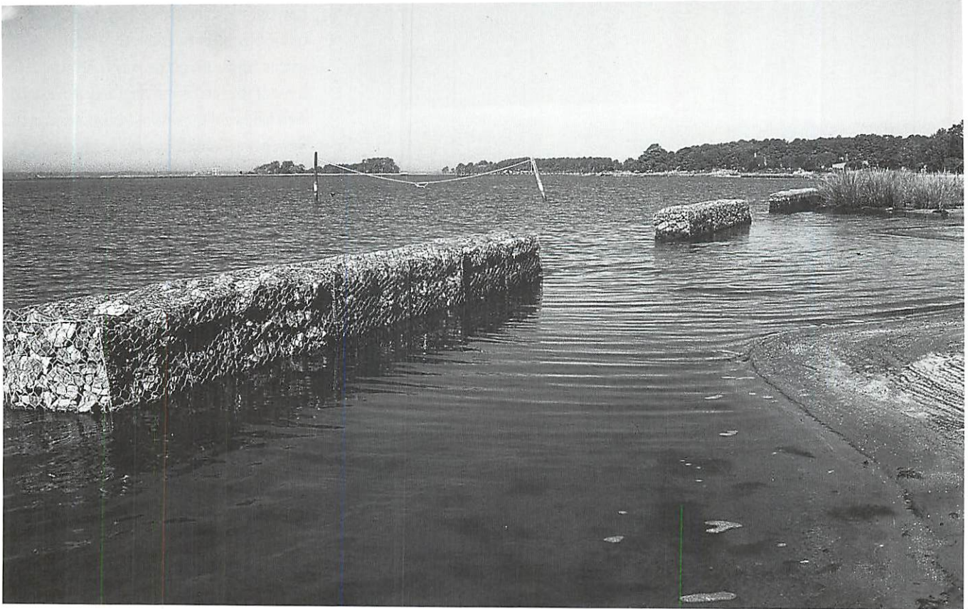
Figure 22. Gabions, showing the wire box to hold the rocks, in a sill-type configuration.
