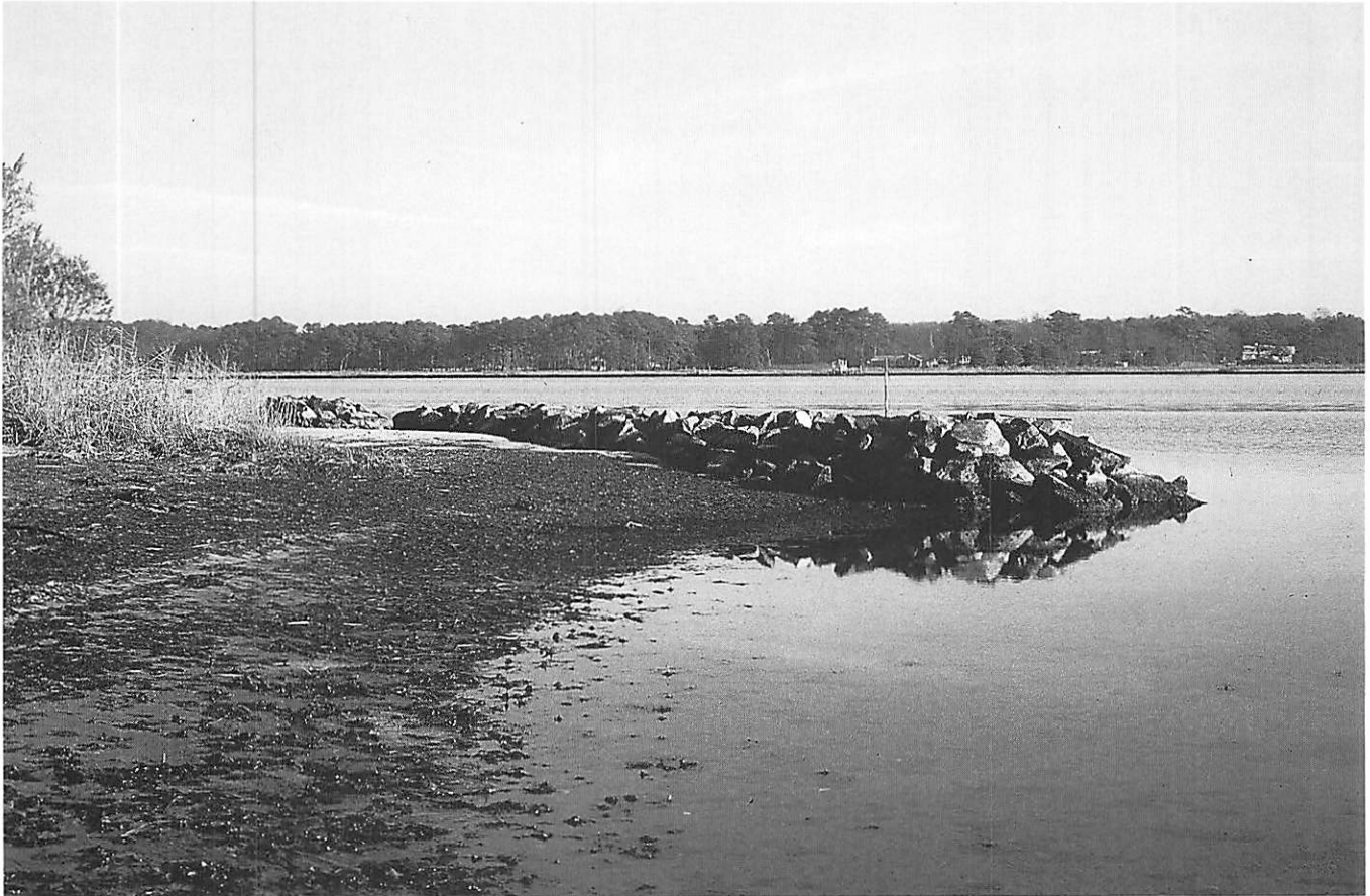
Figure 25. Over time, marsh plants will grow on the sand tombolo behind the breakwater structure.
