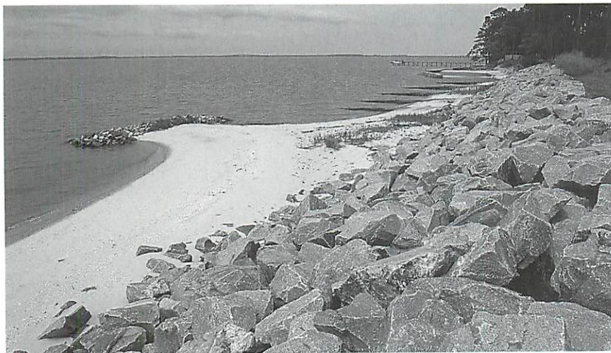
Figure 23, top: A groin field, showing a series of small, wooden groins on a soundside shoreline. Note the crescent sediment design. Figure 24, bottom: An offshore rock breakwater, which has a mature sand connection or tombolo to the shoreline. Groin field in the background.
