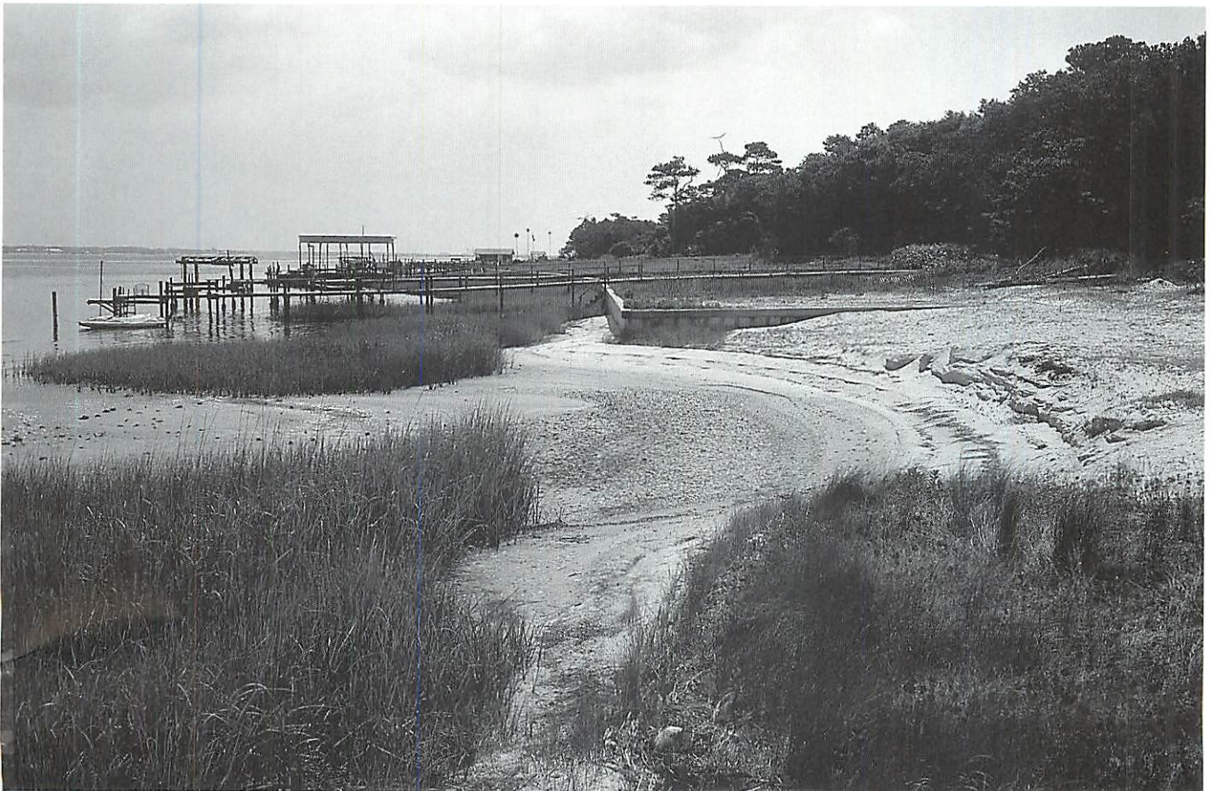
Figure 4. Increased erosion of beach and marsh shoreline adjacent to a bulkheaded lot.
