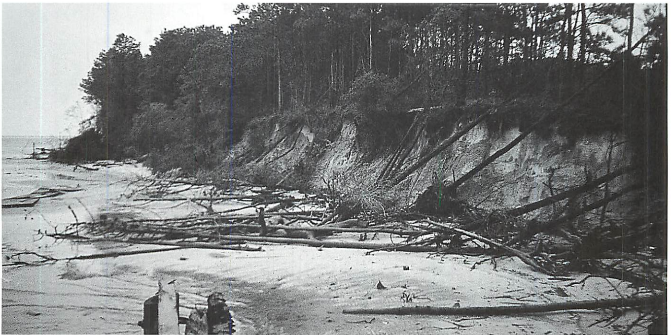
Figure 7, top: Low-bank erosion of a forest. Figure 8, bottom: High-bank erosion of a forest. Note the probable high-tide position.
