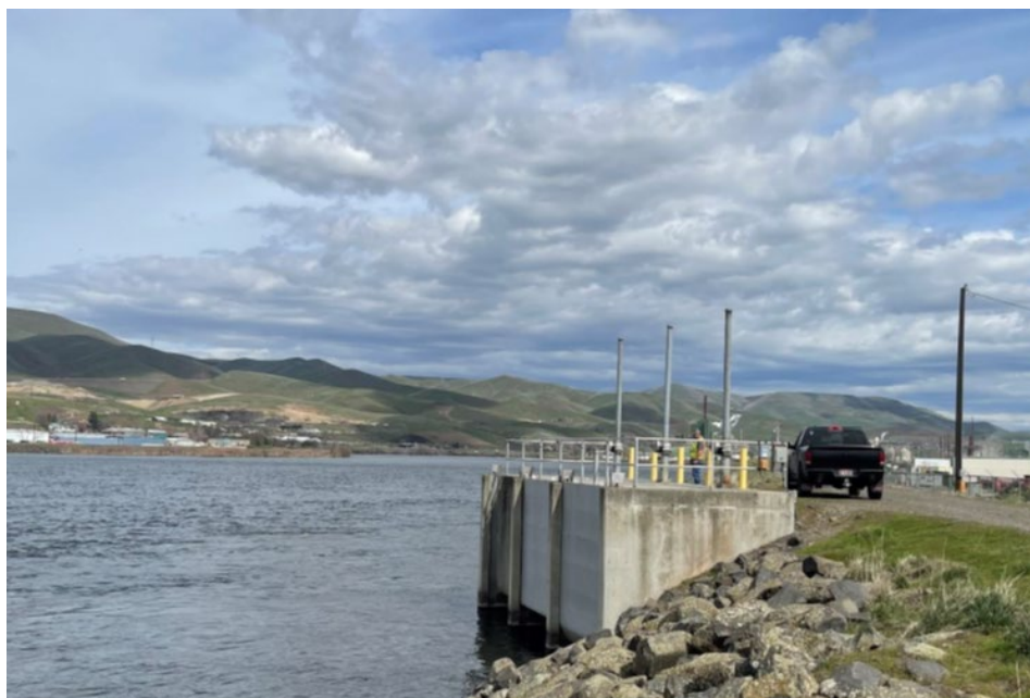
Figure 2. Looking upstream at the Lindsay Creek structure. The bulkheads can be seen at the front (river) side of the structure. The Area 380 structure is nearly identical.
