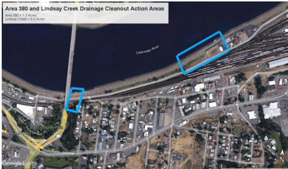
Figure 7. Action areas for the Area 380 and Lindsay Creek culvert cleanouts.
