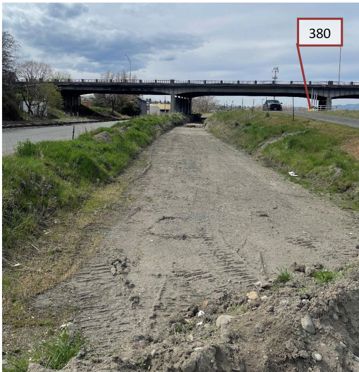
Figure 6. Slurry dewatering area behind the levee at Area 380 drainage.
