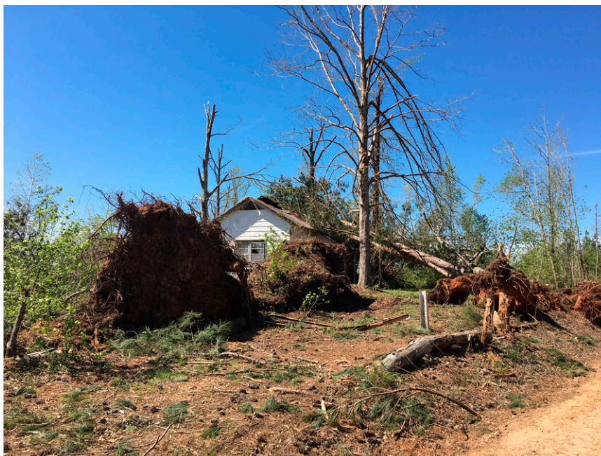
FIG. 5. House with numerous trees fallen onto it just outside the swath of most severe tree damage along Brown Taylor Road.
