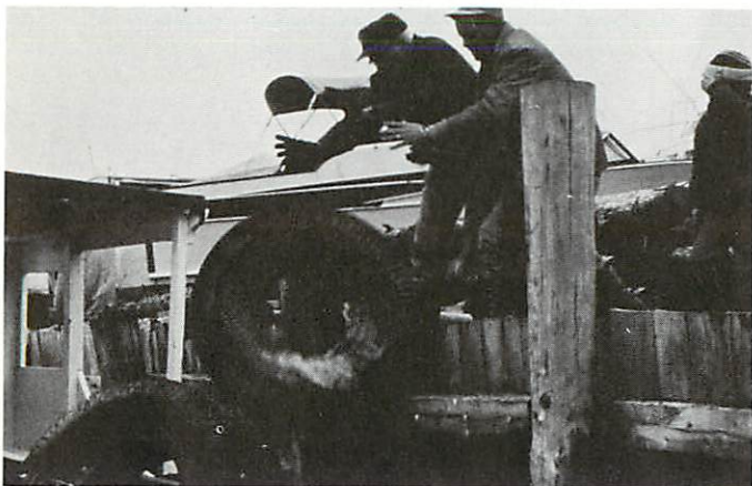
Extension agents assist in construction of artificial offshore reefs.
