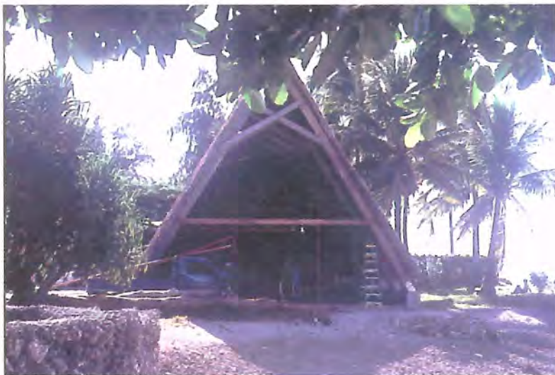
Work-boat construction shed on Majuro.
