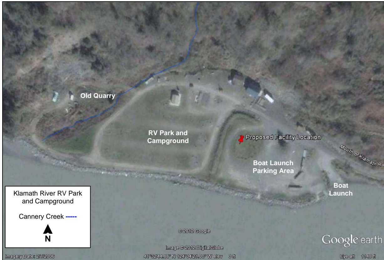
Figure 2. Requa Resort area map displaying proposed fish processing facility location, RV Park and campground, boat launch, and Cannery Creek.
