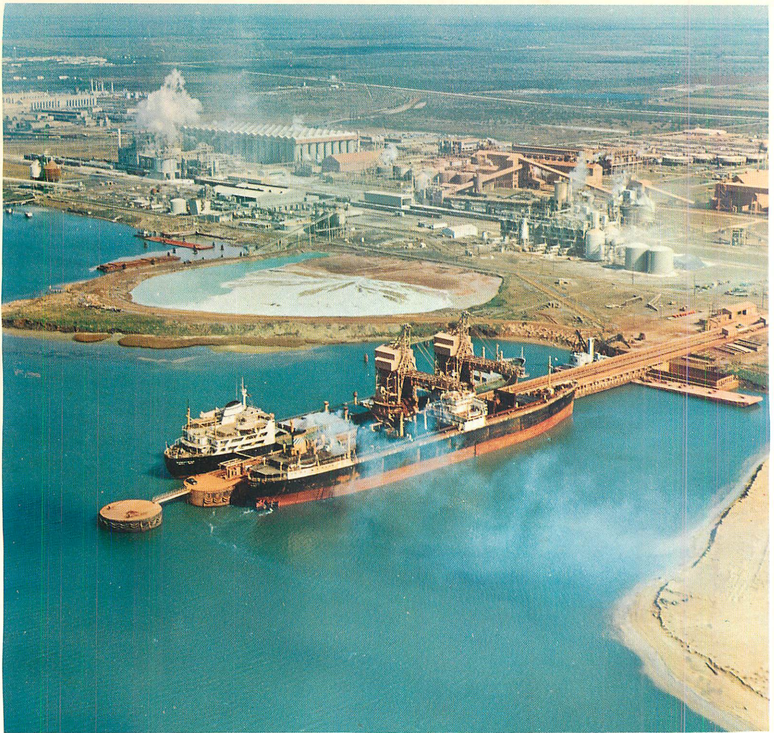
Ocean-going vessels unload bauxite at ALCOA's Point Comfort plant.
