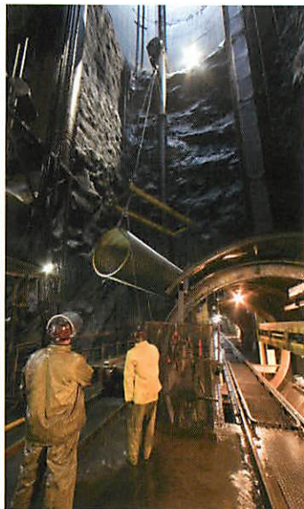
Providence’s combined sewer overflow tunnel has reduced nutrient inputs to Narragansett Bay. Photo courtesy Narragansett Bay Commission.
