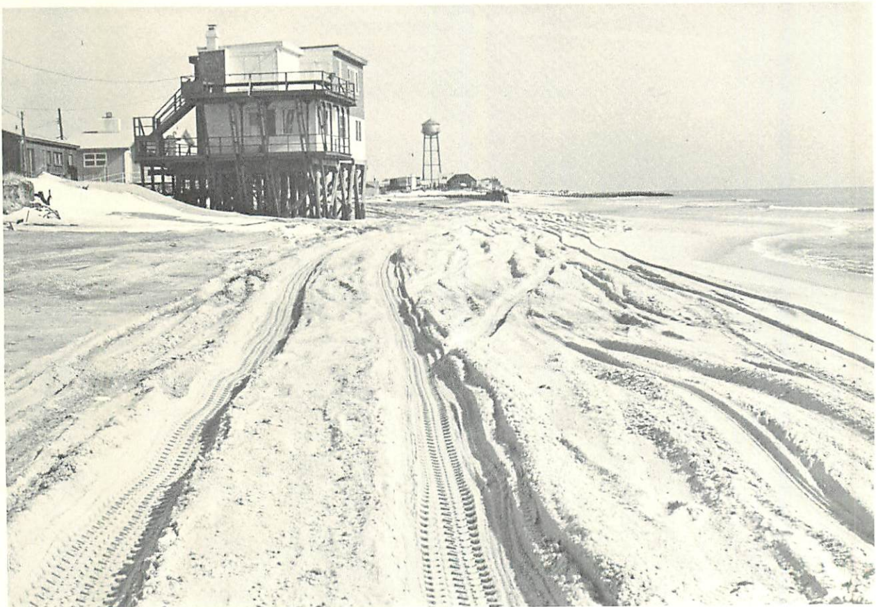
This beach on Fire Island is receding 20 feet per year. Erosion is caused partly by groin in background, built to help protect the water tank.
