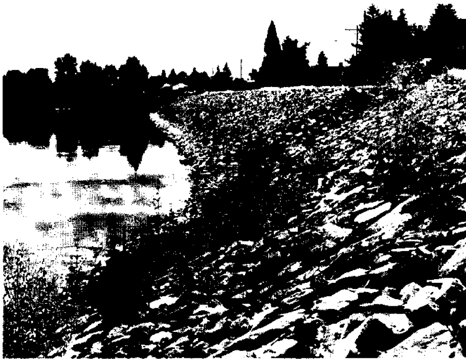
Riprap is a common streambank erosion-control method, but it may adversely affect both aquatic and riparian habitats.
