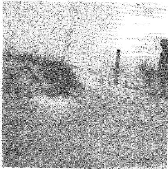
Fig. 42. A sand fence used to fill a gap in the fore dune line is now almost completely covered by sand. Sea oats are well-established after two years.
