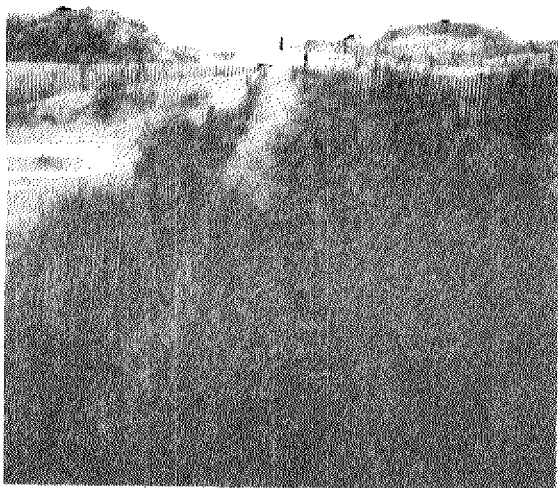
Fig. 46. Arrangement of sand fences to protect and encourage panic grass growth.
