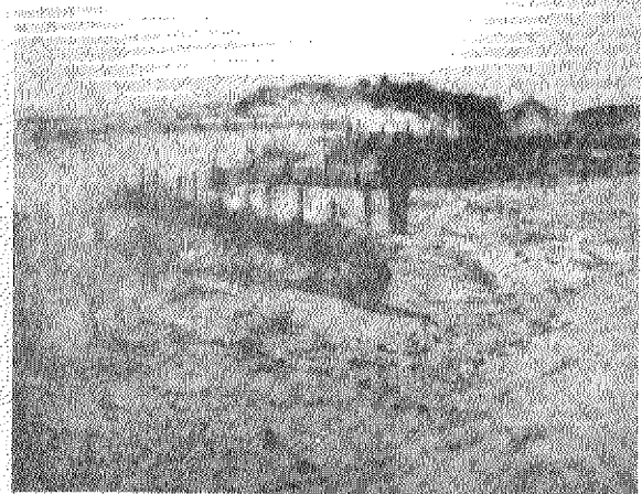
Fig. 47. Sand fences positioned across direction of prevailing wind, also some plantings in this eroded dune field.
