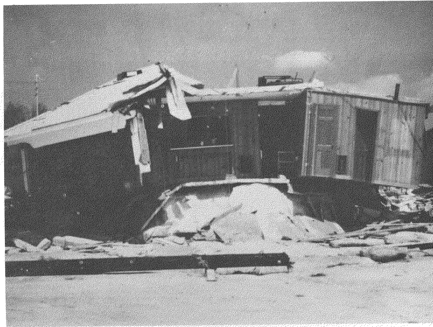
Figure III-9. Waves washed the supporting sand from under the slab on grade, causing the slab to fracture and the house to fall. Hurricane Eloise (9/75)
