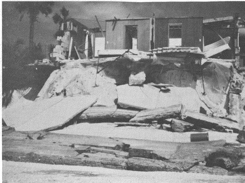
Figure III-9. Waves washed the supporting sand from under the slab on grade, causing the slab to fracture and the house to fall. Hurricane Eloise (9/75)
