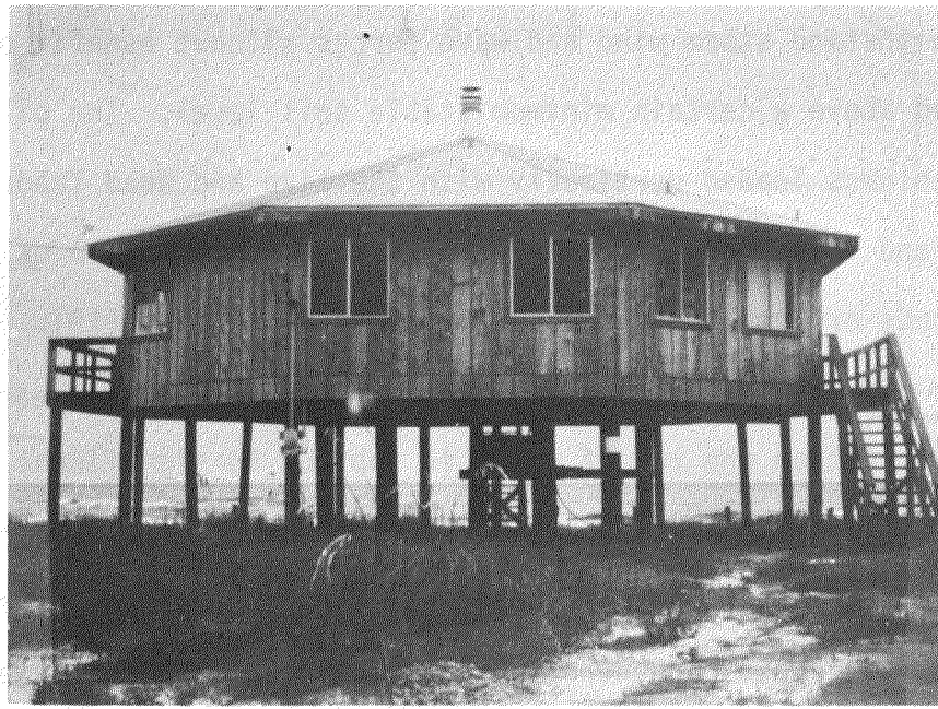
Figure IV-7. Typical Pile Supported Structure (43).
