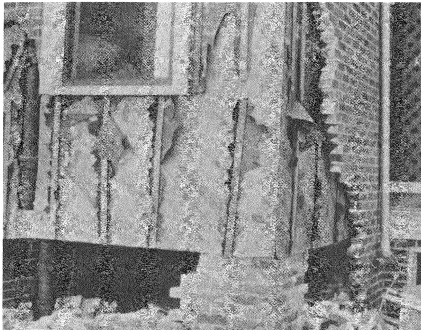
Figure III-17. Hurricane Damage to Brick Veneer Siding Resulting From Wave Action. Diagonal Sheathing Provided Excellent Rigidity As Well As A Good Tie Between Wall and Floor Framing (4).
