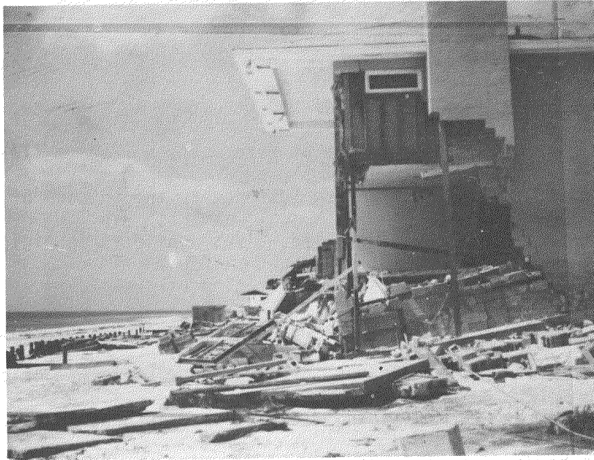
Figure III-15. Failure of Corner Walls Due to Wave Action and Loss of Support
