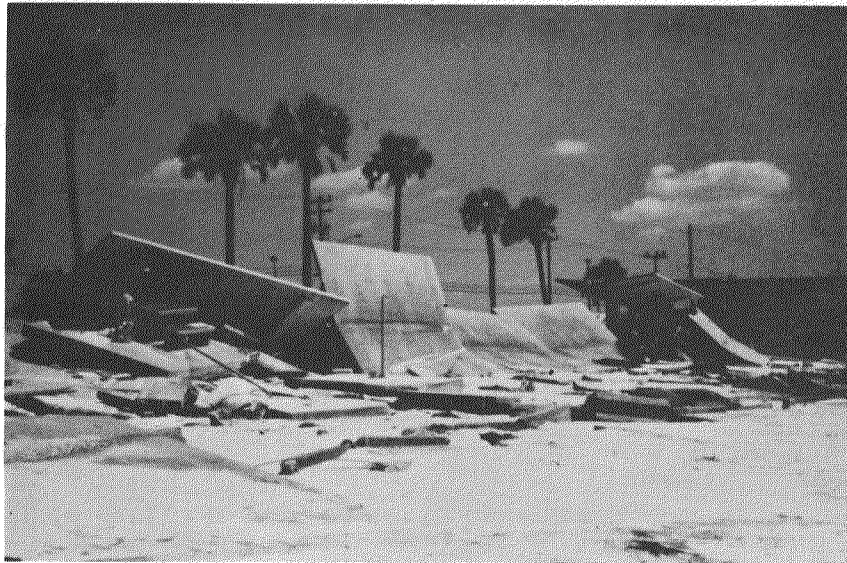
Figure III-7. Structural Failure Due to Wave Action. Roadside Rest Area, approximately 250 feet from the Shoreline, Panama City Beach, Florida, Hurricane Eloise, Shallow Foundation, No Piling (9/75)
