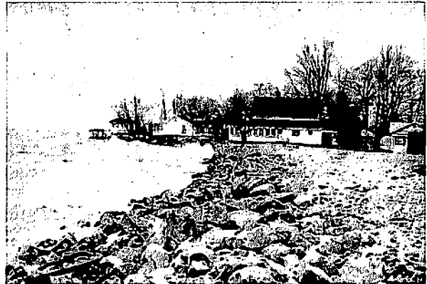
Figure 22. Tawas Point Coast Guard Station, April 25, 1976.
