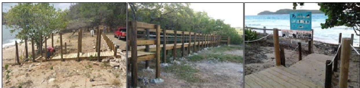
Figure 35. Examples of elevated boardwalks and delimitation of sensitive vegetation areas while allowing public access to beaches (Photo source: Protectores de Cuencas)
