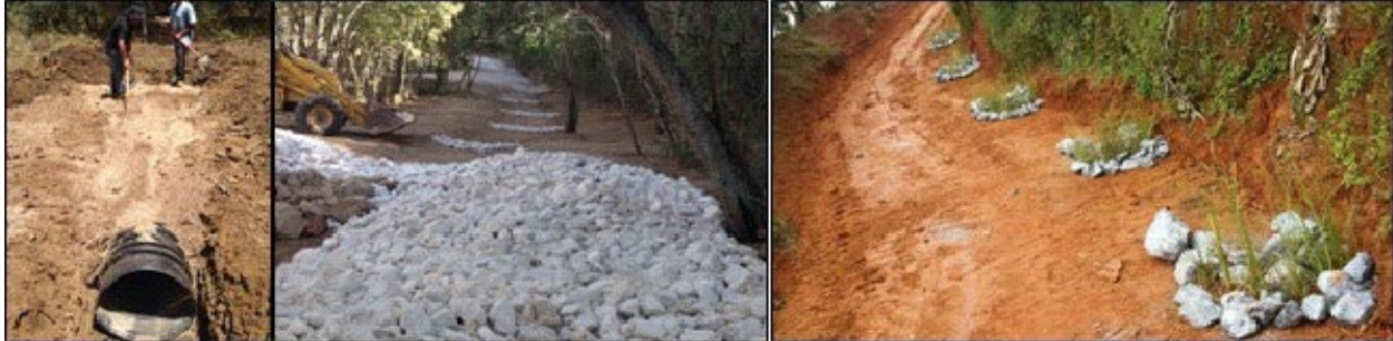
Figure 33. Dirt road stabilization in Puerto Rico (Photo source: Protectores de Cuencas)
