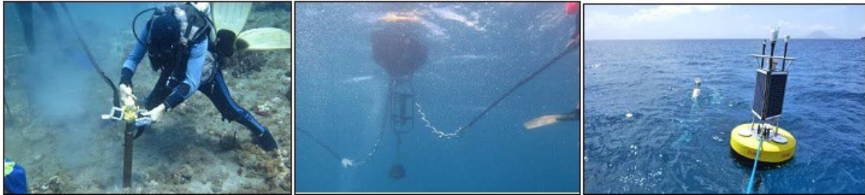
Figure 7. Coral Reef Early Warning System buoy installation (Photo source: NOAA Atlantic Oceanographic and Meteorological Laboratory)
