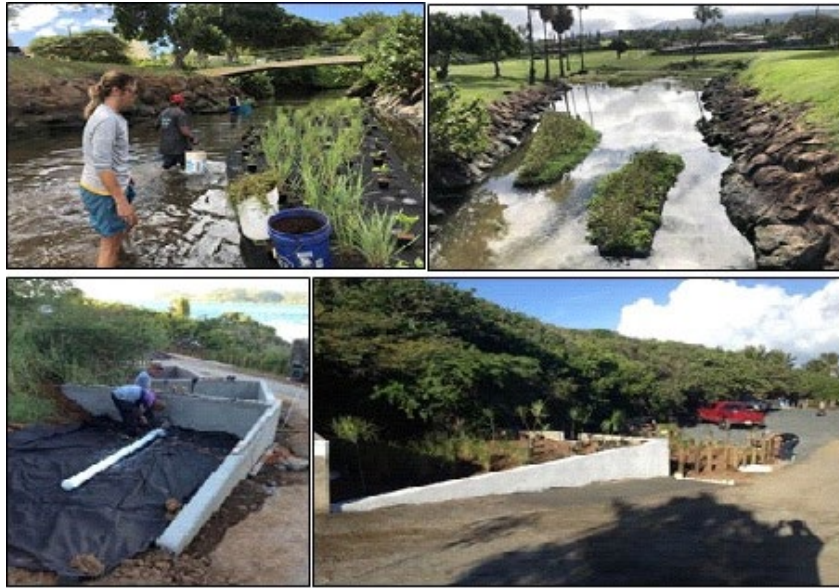
Figure 40. Examples of wetland construction (left) and completion (right) (Photo source: West Maui Ridge to Reef [upper row]; Protectores de Cuencas [lower row])
