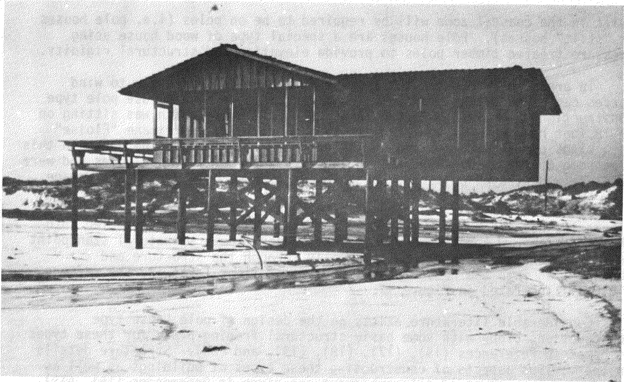
Figure 16. Pole house which survived Hurricane Eloise.
