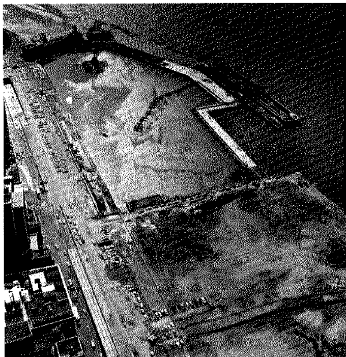
Figure 3b. September 1973—completed bulkhead before sand pumping started
