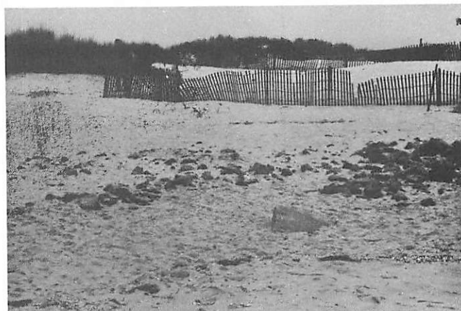
Using snowfences to hold sand. These fences have not been carefully placed or properly maintained.
