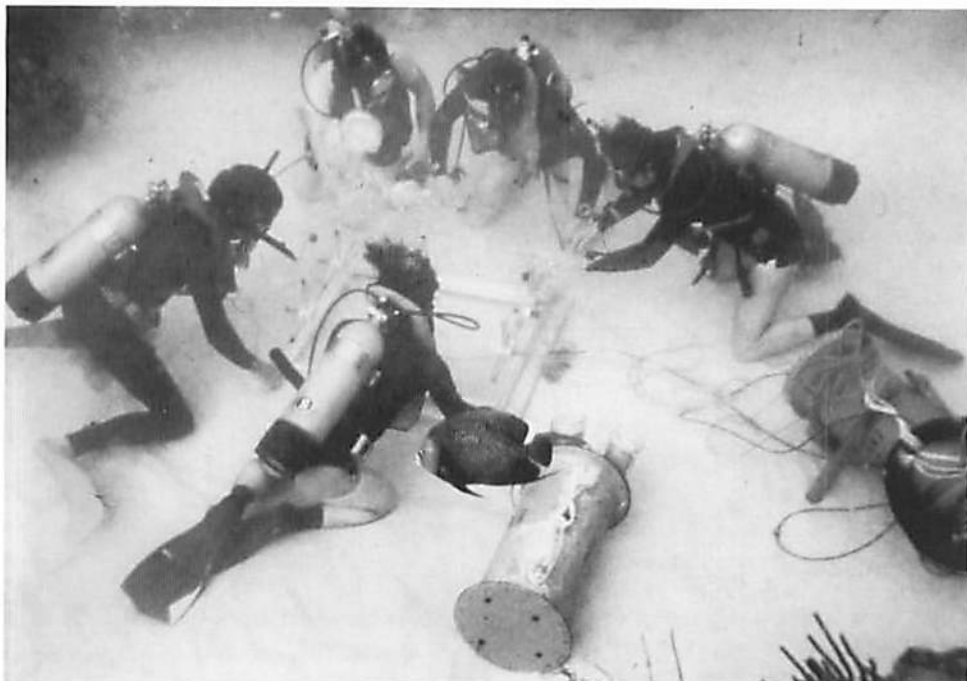
Student project team emplaces base and acrylic dome of chamber for holding a community of marine algae. The power supply cylinder is in the center foreground. The instrument case is to the right. Freeport, Bahamas, March, 1974.
