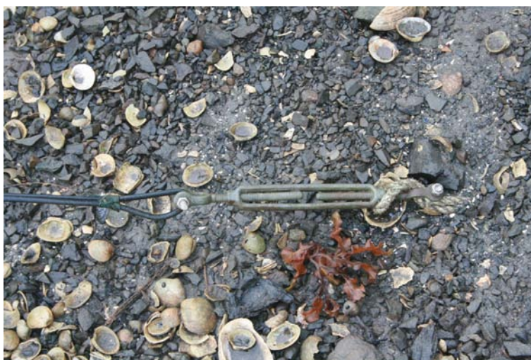
Figure 10. Anchor formed by bolting a turnbuckle to a rock.
