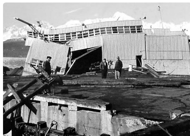
Several tsunamis hit the Seward waterfront after the 1964 Alaska earthquake. This photo shows damage at the site of the present SFOS Institute of Marine Science Center.
