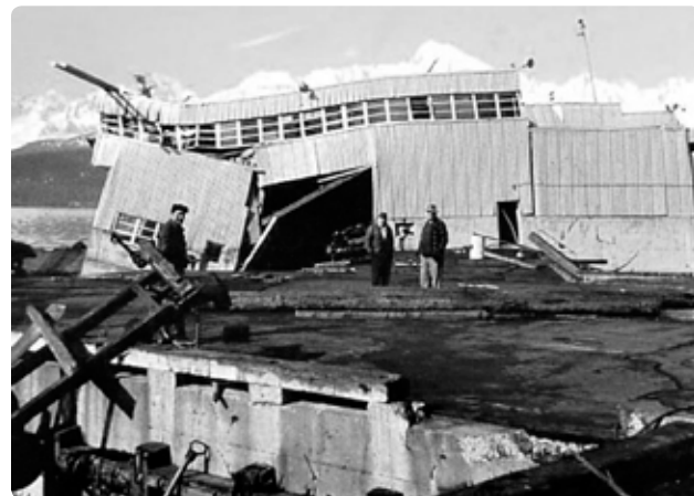
Several tsunamis hit the Seward waterfront after the 1964 Alaska earthquake. This photo shows damage at the site of the present SFOS Institute of Marine Science Center.
