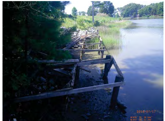
The remains of an old dock could be replaced with a living shoreline to stop the undercutting of the bank.
