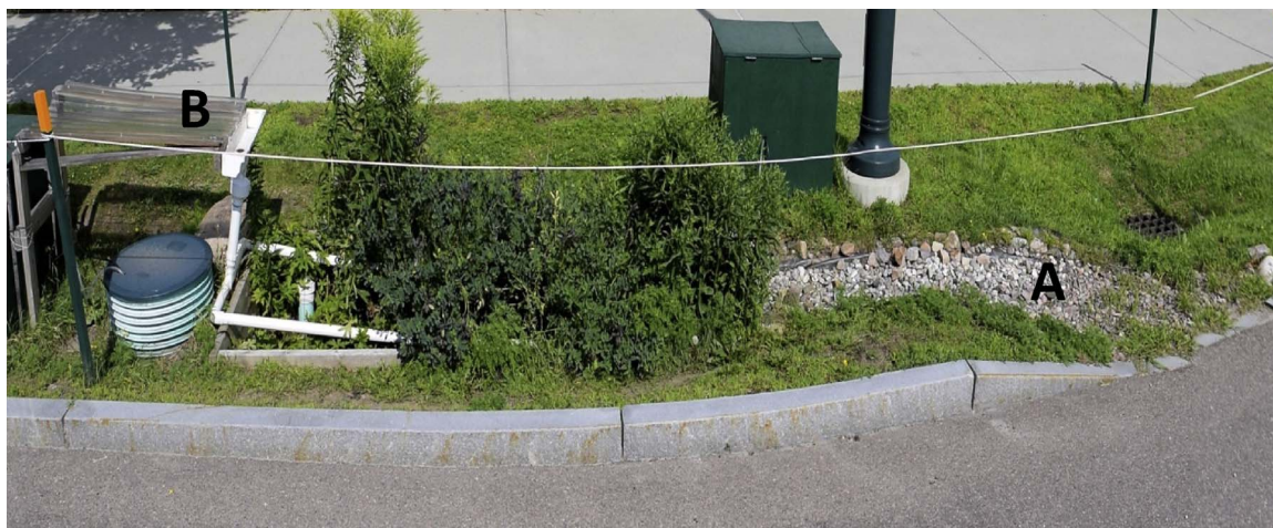
Fig. 1. Bioretention cell at the University of Vermont, Burlington, USA. The cell receives road runoff via curb cuts along the road. (A) Shallow rock-line inflow swale, underlain by high-density polyethylene (HDPE) plastic, conveys runoff into the cell’s weir. (B) Rainpan and attached PVC precipitation-distribution pipes. The rainpan is installed outside of the cell. Rainwater from the corrugated pan drains into gutters, vertical downspouts, and to pipes that run horizontally along the length of the cell and contains perforations at the bottom to deliver water evenly across the cell. Photo credit: Lindsay Cotnoir.
