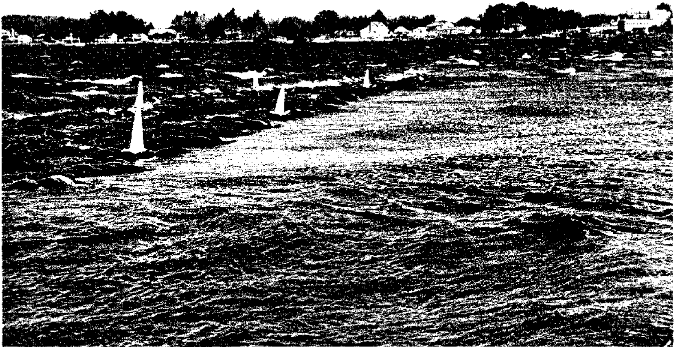
The Great Bay Marina floating tire breakwater in action on a brisk and breezy November day.
