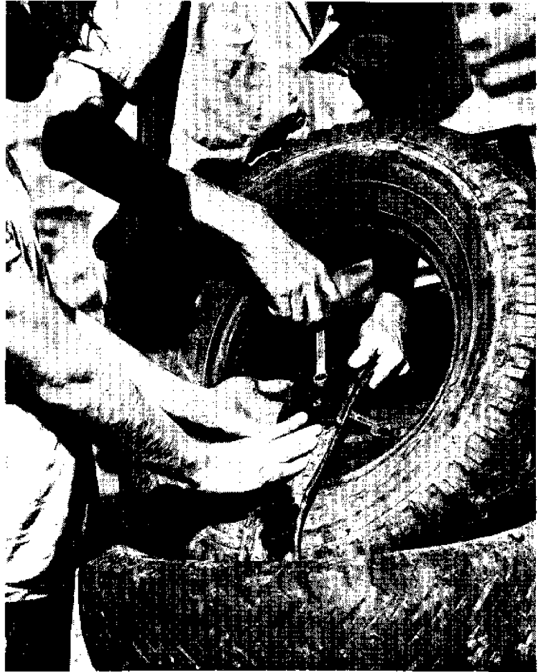
The floating tire breakwater installed at the Great Bay Marina in Newington, New Hampshire, in September, 1976, was bound together with conveyor belt edging material. Three 3/8-16 bolts per fastening were used to secure the bonds.
