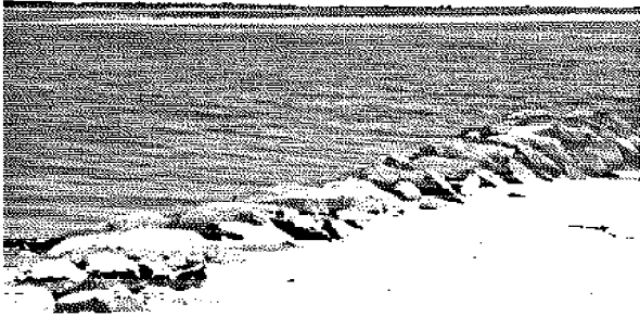
Photo #41. Sta. VIII. Groin 14, displaying sand accumulation on SW side of groin and erosion on NE.
