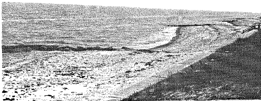
Photo #14. Sta. V. Southernmost 5 groins, looking south. Photo displays sand capture on northern side of groins in June 1982.
