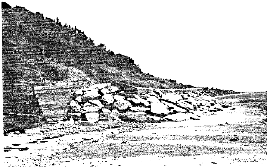
Photo #9. Sta. IIIa. Seawall with stone apron, looking northeast.
