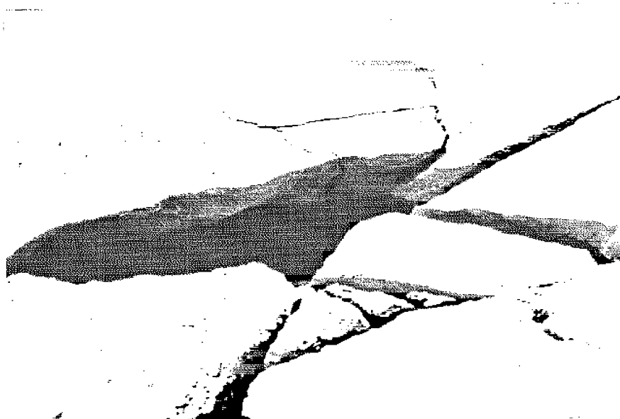
Photo #27. Sta. VI. Cracked revetment between groins 10&11, showing space where sand has been eroded beneath the concrete.
