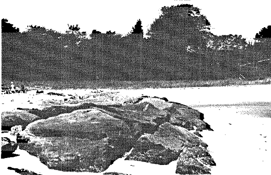
Photo #38. Sta.VIII Groin 8, looking shoreward, displaying sand accumulation on southwest side of groin, nearly overtopping structure.
