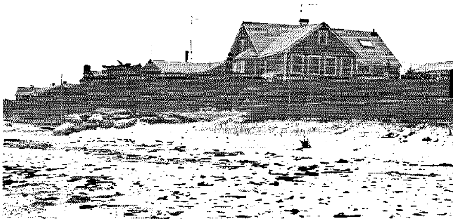
Photo #16. Sta. Va. Northern end of seawall between second and fifth groins. Extent of erosion of unreinforced bluff can be seen to the right of the boulders.
