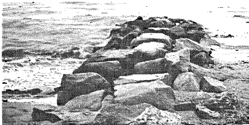
Photo #15. Sta. V. Groin displaying sand accumulation on southern side of structure in January, 1983.
