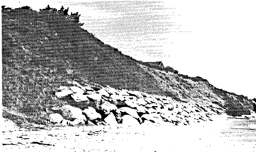
Photo #12. Sta. IIIc. Concrete seawall with boulder apron & cliff vegetation for increased stability; looking northward. Note increased landward migration of cliff immediately north of seawall.
