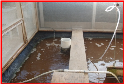
Picture 3: RW drain and filter pipe.
