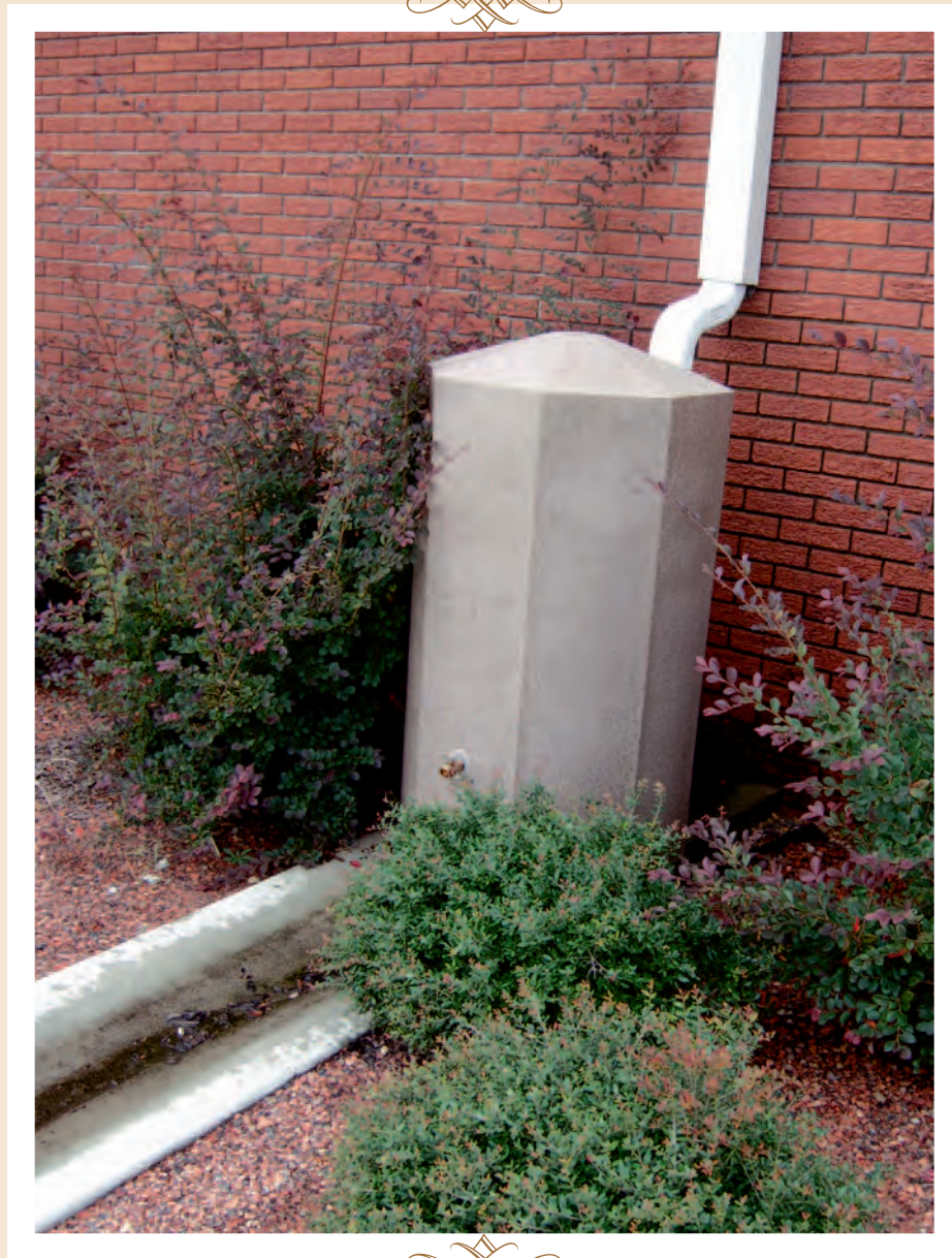
An example of a rain barrel located at Coastal Carolina University's Burroughs and Chapin Center for Marine and Wetland Studies in Conway, SC. The barrel collects stormwater from a gutter downspout and has an overflow mechanism that activates when the barrel is full.
