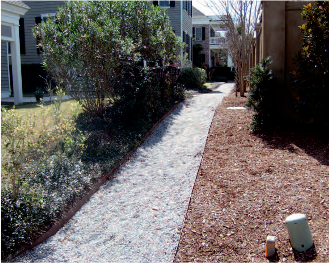
An example of a pervious landscape, including a crushed stone walkway, natural buffer areas, and a mulch area. These landscape features allow for stormwater to flow and filter into the soil rather than running off into the street.
