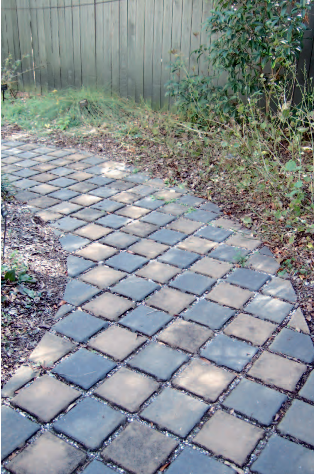
An example of an attractive paver sidewalk located at the Center for Sustainable Living at 113 Calhoun St. in downtown Charleston, SC. Pavers allow for stormwater to flow and filter into the soil rather than running off into the street.
