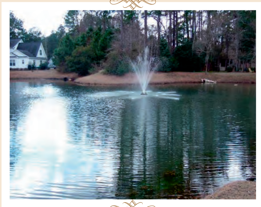
An example of a fountain aeration system installed in a stormwater pond.
