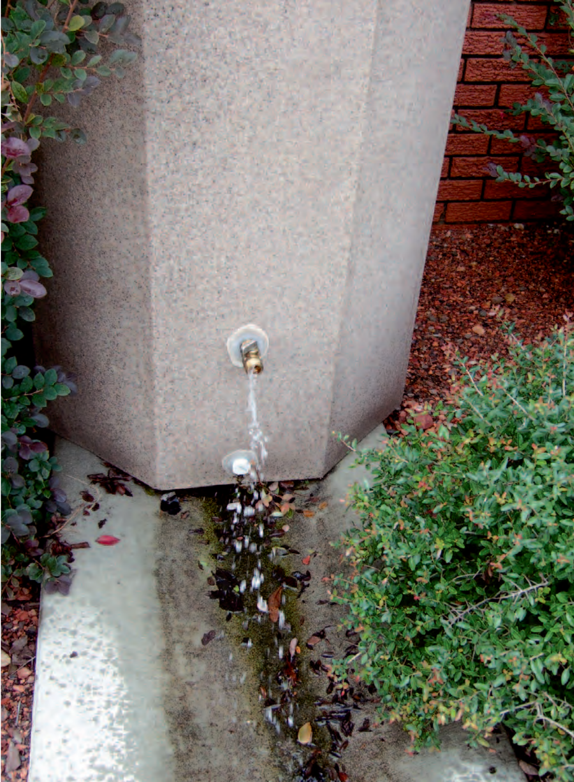
The rain barrel collects stormwater from the rooftop, which can be controlled to irrigate your yard during dry conditions.
