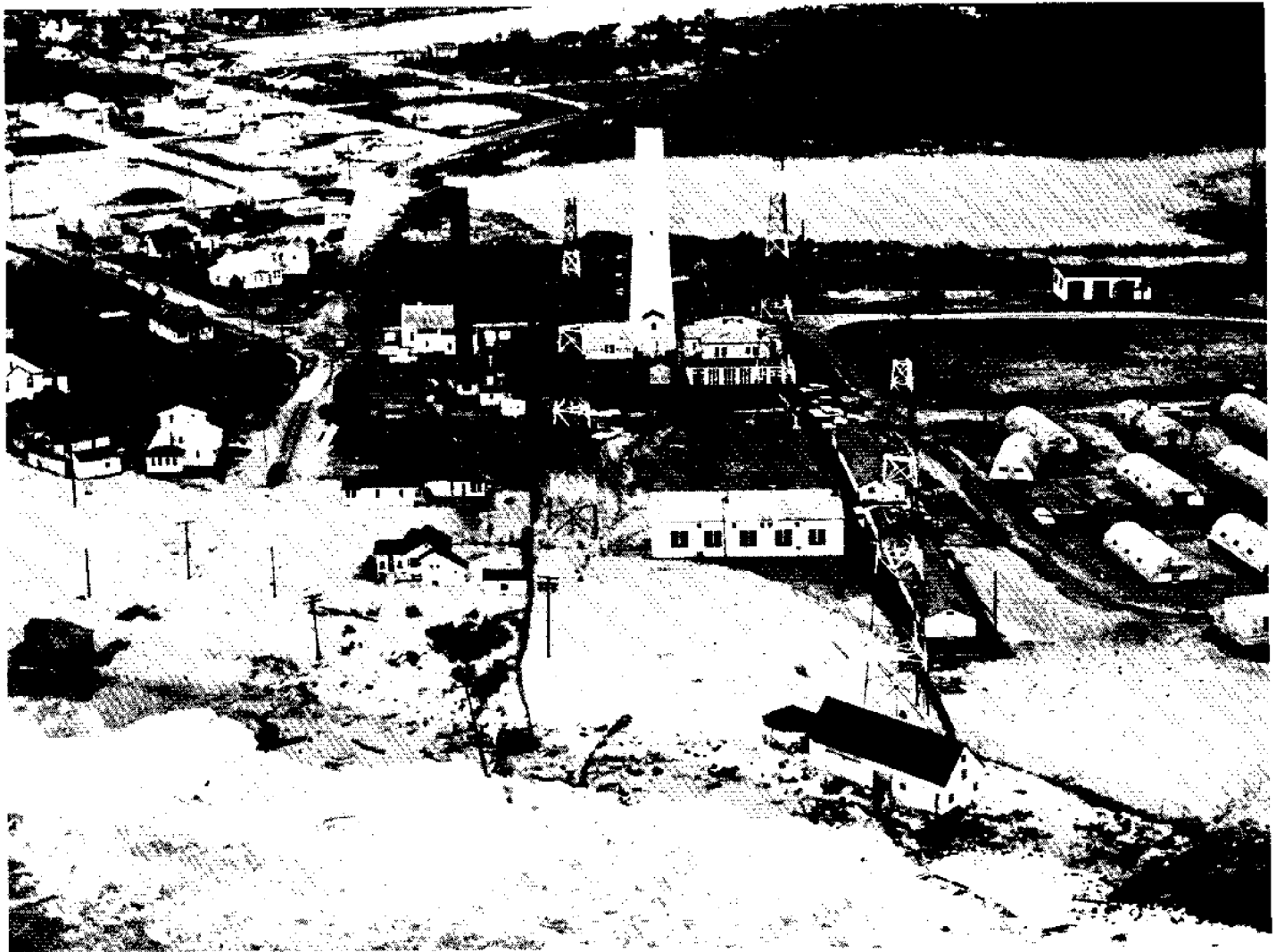
Figure 26. View north at Cape May Light Station, Cape May Point, 9 March 1962. The white arrow shows the line of maximum wave attack 120 m (400 ft) landward of mean high tide line. (Courtesy of US Coast Guard Headquarters, Washington, DC)
