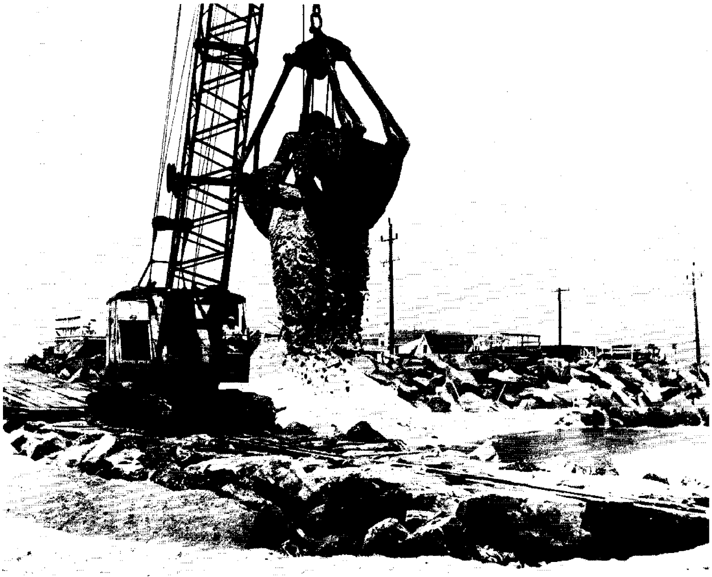
Figure 32. Strengthening timber and woodpiling groin with rip-rap, Sandy Hook, September 1960. Rip-rap was removed from seawall to build a ramp for the power shovel. After rip-rap blocks were put on both sides of the groin, stockpile sand was dumped around groin and rip-rap. (Photo by W. Yasso)
