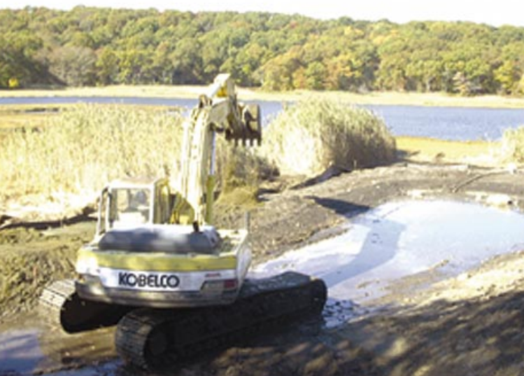
Construction on the Narrow River project begins.
