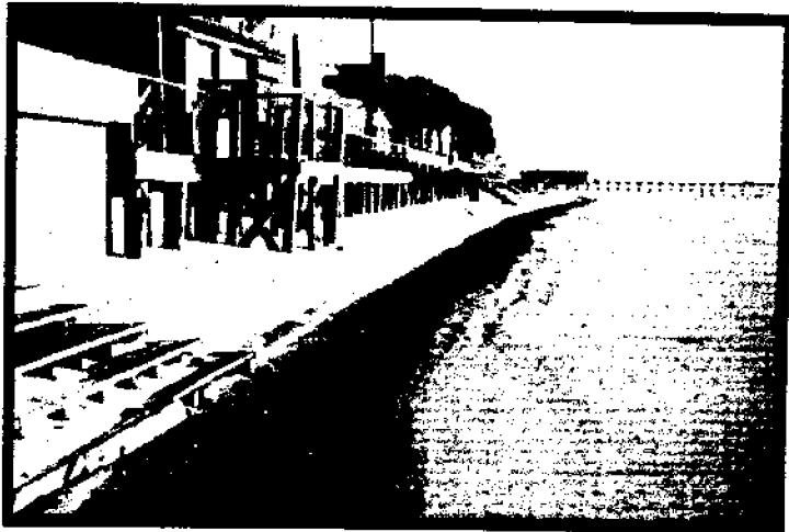
Scouring caused by presence of seawall; the seawall doesn't cause large-scale erosion, but does accelerate erosion of high tide beach by blocking exchange of sand from dunes.
