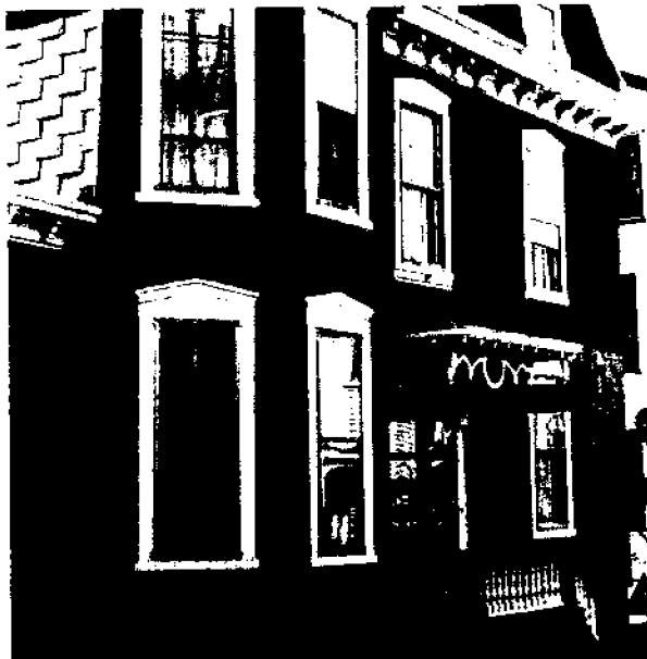
Asbestos shingle siding is an example of an inappropriate modification to an otherwise high-scoring building.
