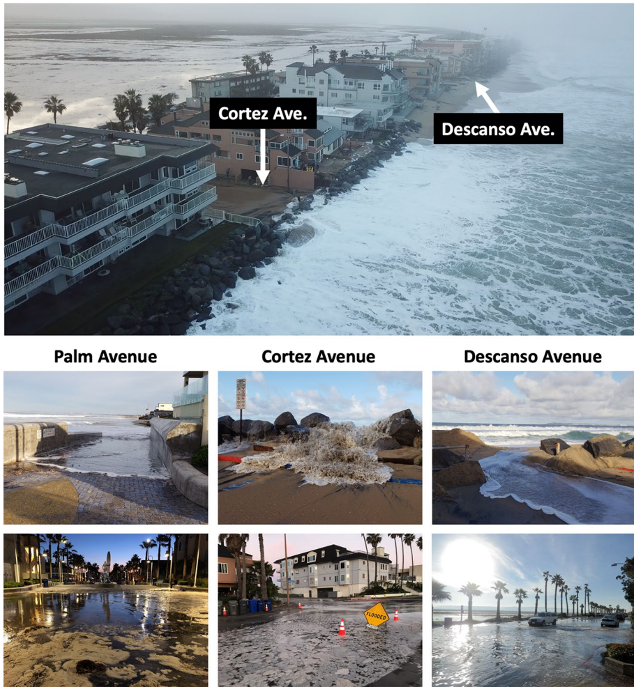
Fig. 2 (Upper) South Imperial Beach during a moderate flood on 18 Jan 2020. LiDAR scans of the swash zone (discussed in F20) were collected from a condominium balcony at the seaward end of Cortez Ave (Arrows). (Middle) Entry points for street flooding include: directly through public access through the berm at Seacoast Dr, over riprap rock at Cortez Ave, and through an access point in the seawall at Palm Plaza. (Lower) Flooding occurs landward of these entry points
