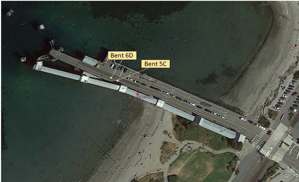
Figure 9. Emergency project elements at the Edmonds Ferry Terminal.
