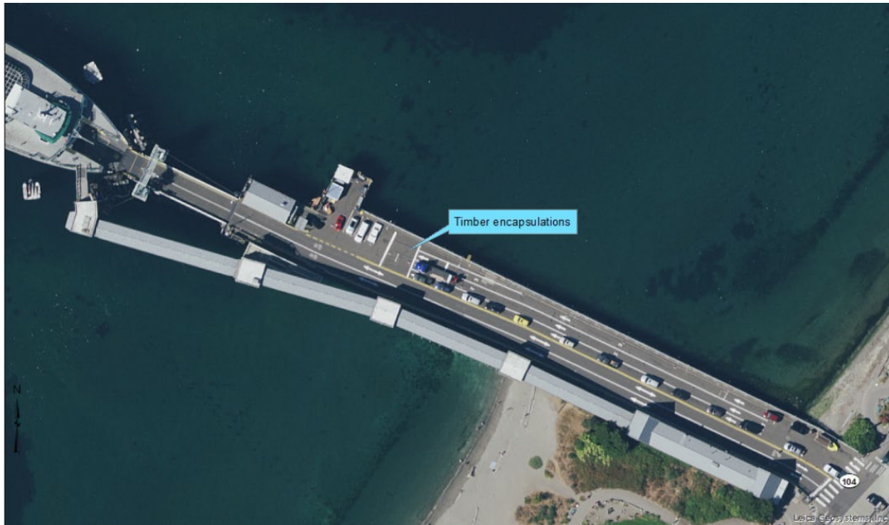
Figure 8. Project elements at the Edmonds Ferry Terminal.
