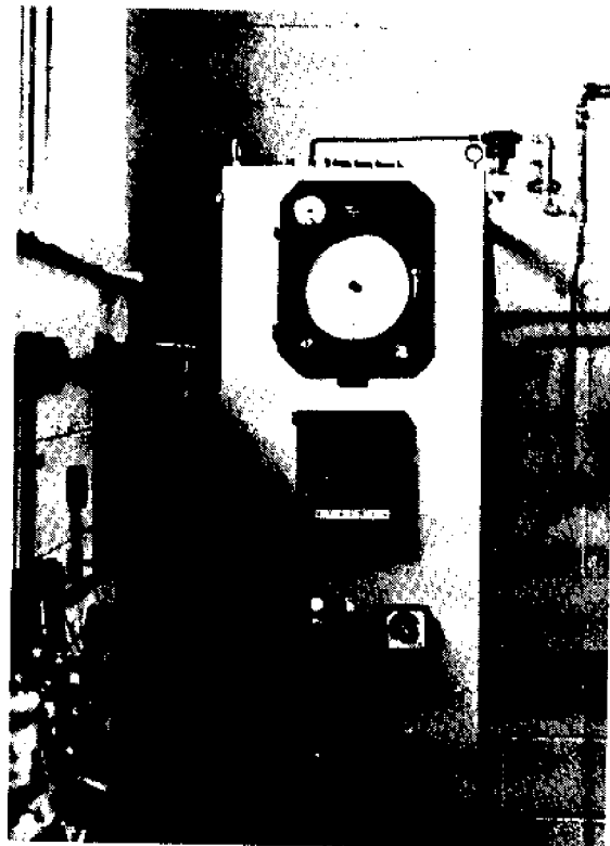
Figure 4. Close-up of panel controls for semi-automatic operation of retort basket.
