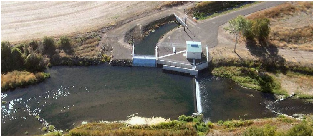
Figure 8-1. Aerial view of the Garden City-Lowden 2 water diversion on Walla Walla River near Touchet, Washington (Notes: River flow is from left to right. The bankline screen is located at the head end of the canal, just upstream of the spillway and adult ladder exit.)
