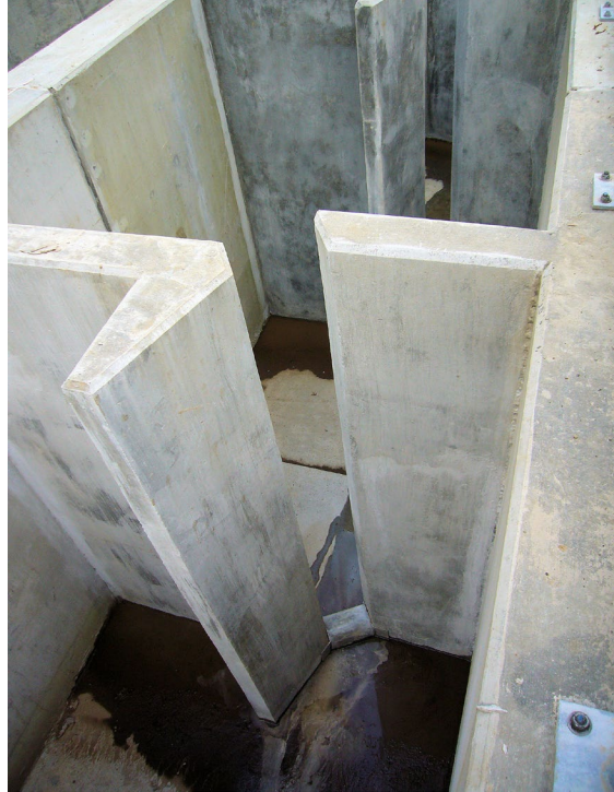
Figure 5-4. Oblique view of a vertical slot ladder baffle when dewatered
