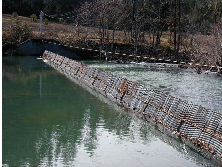
Figure 6-6. Elk Creek Dam picket weir (Elk Creek, Oregon)
