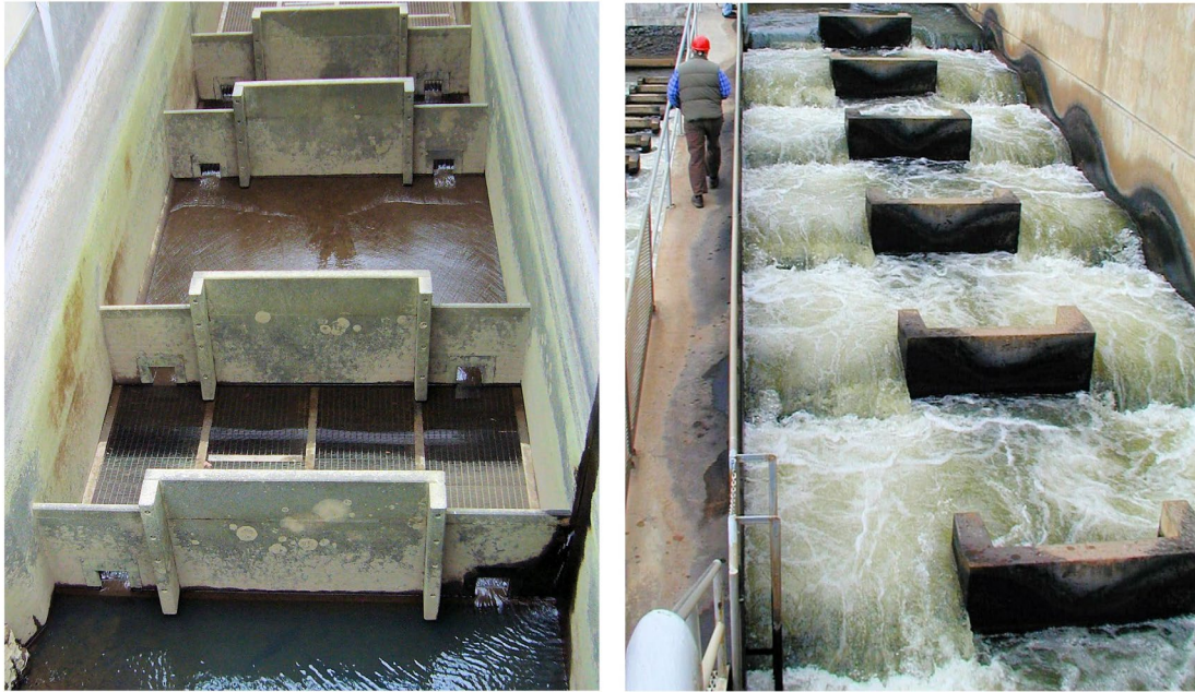
(a) Looking downstream
