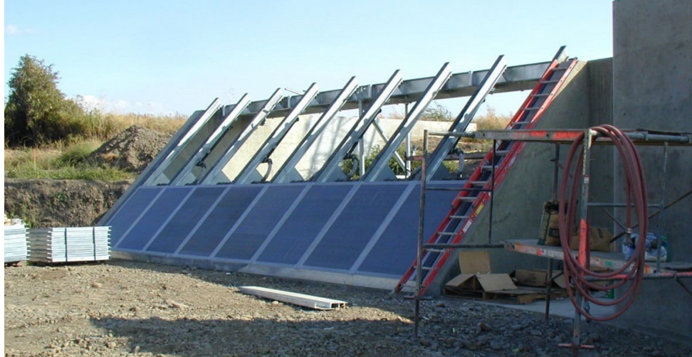
Figure 8-2 Bankline screens at the Garden City-Lowden 2 diversion on the Walla Walla River near Touchet, Washington, under construction
