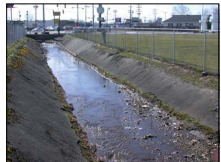
Figure 28. Channelized section of Cascade Creek in Cascade Creek subarea 7
